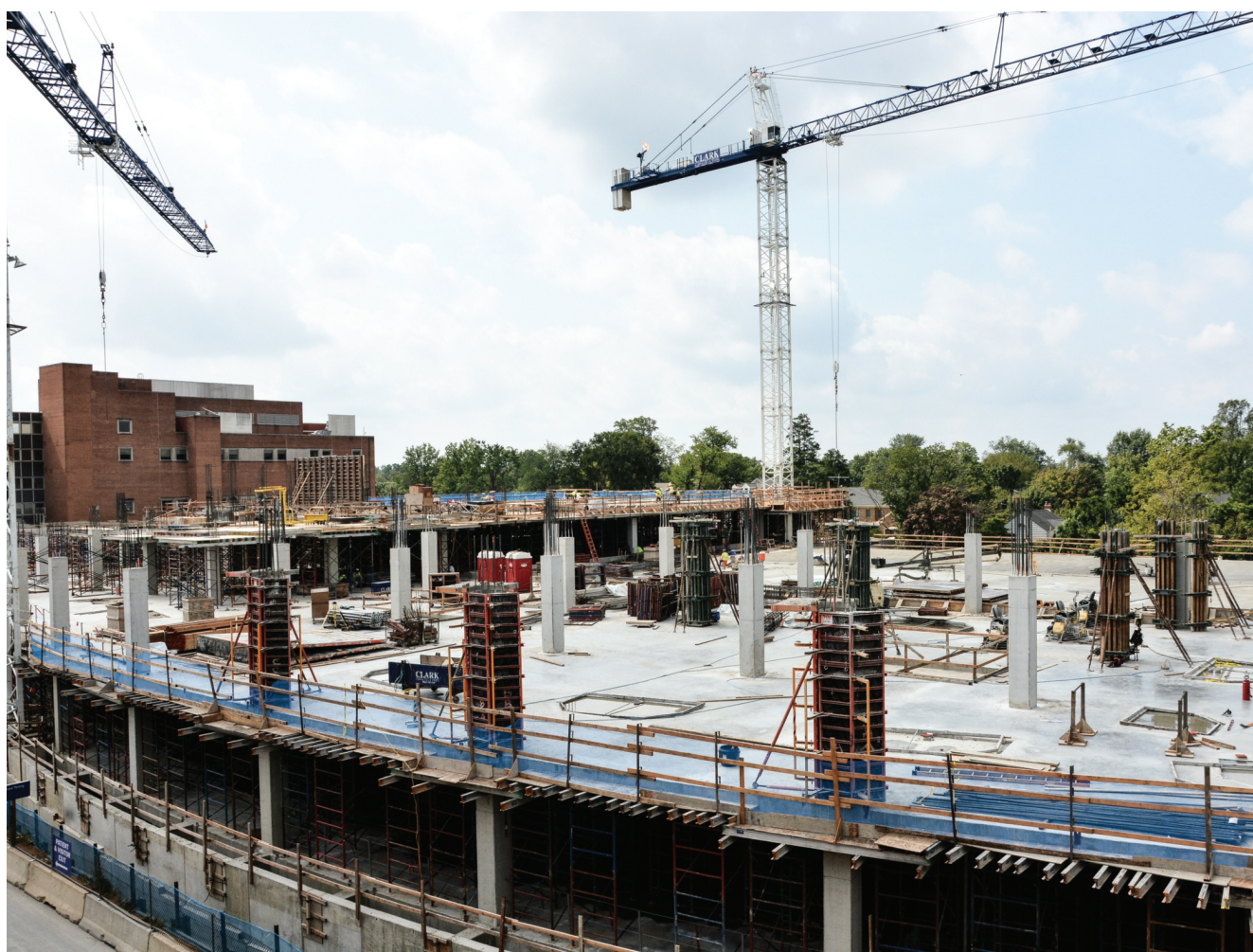
Suburban's new building is due for completion in 2019/early 2020
