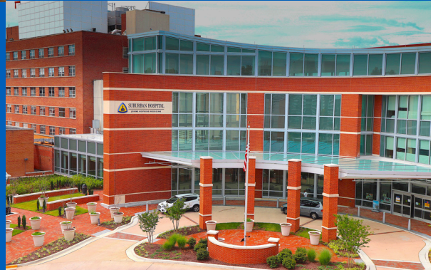
▼ Suburban Hospital Bethesda, Maryland
